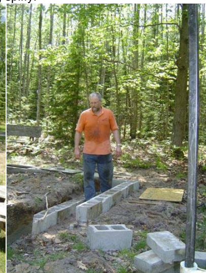
Kevin Dovovan rebuilds earthdog liners with concrete block
